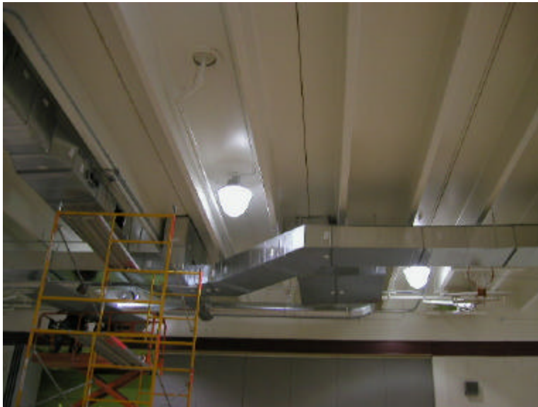
Two views of new roofing and new ductwork installation in gymnasium.
